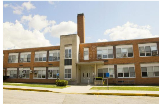
Figure 8: State of the art school building
